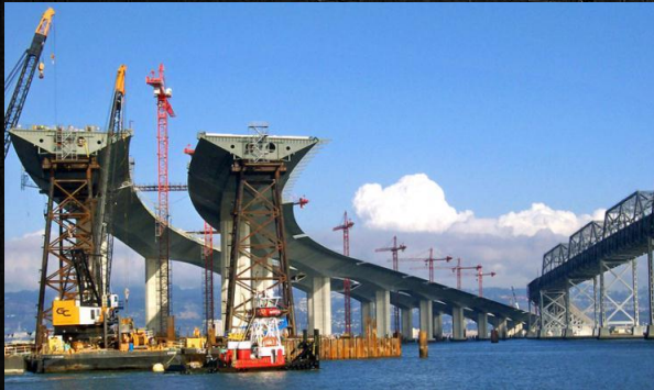
Oakland Bay Bridge – Touchdown Structure
