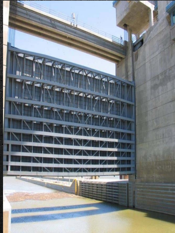
4 Lubron TF slot-loader track roller bearings Olmsted Bulkhead Maintenance Gate Ohio River, Illinois (2006)
